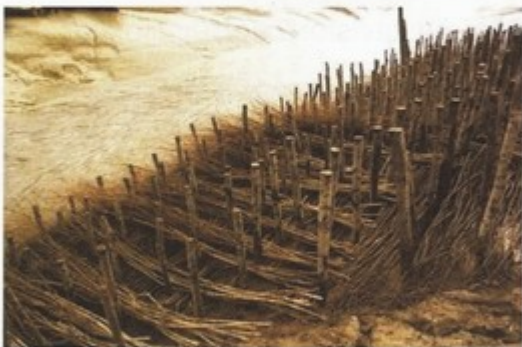
Trial construction: more faggots than you can shake a stick at.
