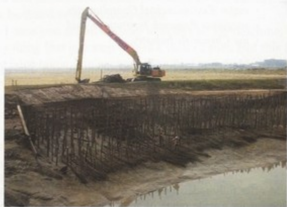
22m reach Komatsu and two faggoters shows scale of works.
