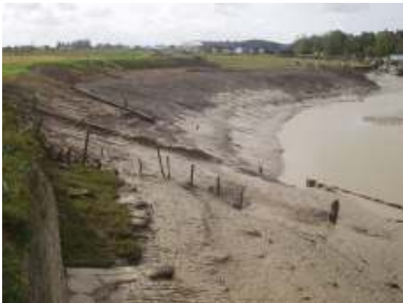
Photograph 14: Mattress at end of construction
