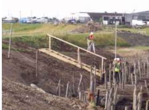
Photographs 10-11: Completion of stake matrix and placement of faggots with temporary step access
