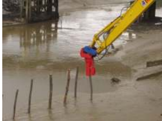
Photograph 8-9: Placement of the timber stakes using placing tool
