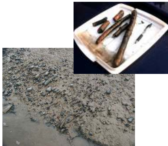
Photograph 5-7: Ancient hazel faggot bank revetment upstream of Monk Bretton Bridge
