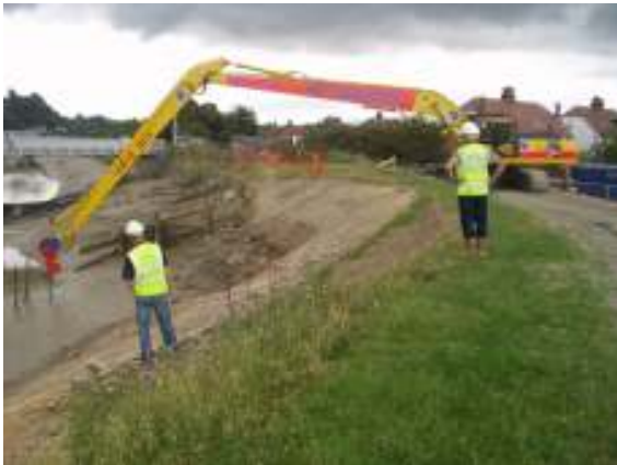
Photograph 8-9: Placement of the timber stakes using placing tool
