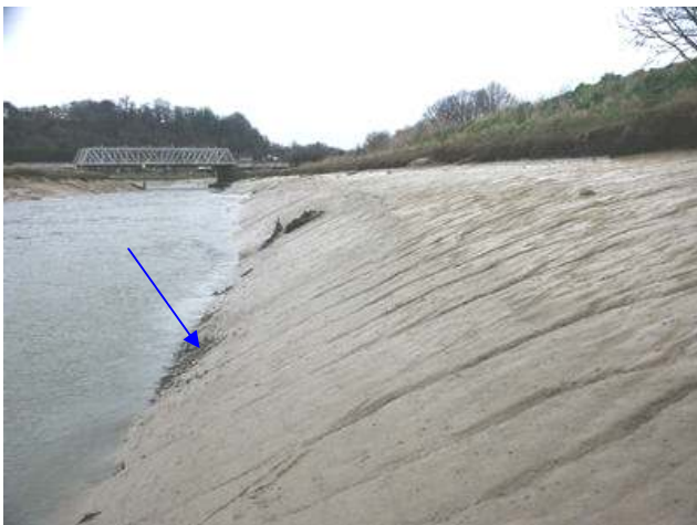
Photograph 5-7: Ancient hazel faggot bank revetment upstream of Monk Bretton Bridge
