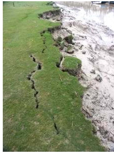
Photo 4: Deconstructing bank margin
