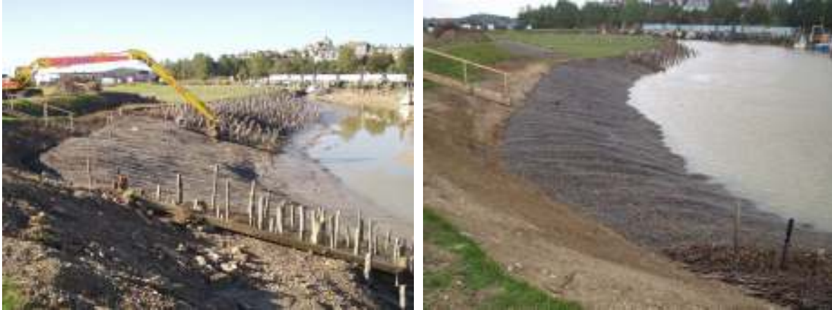
Photograph 12-13: Mattress with netting installation
