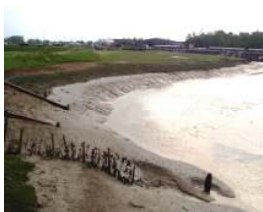
Photograph 15: 12 months post completion
