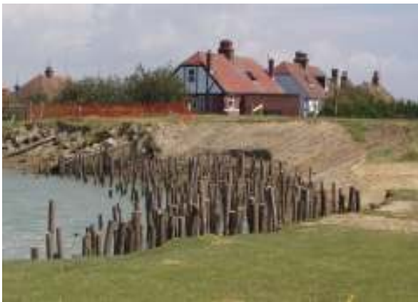
Photographs 10-11: Completion of stake matrix and placement of faggots with temporary step access
