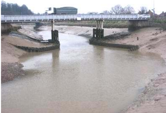
Photo 1: Monk Bretton Bridge
