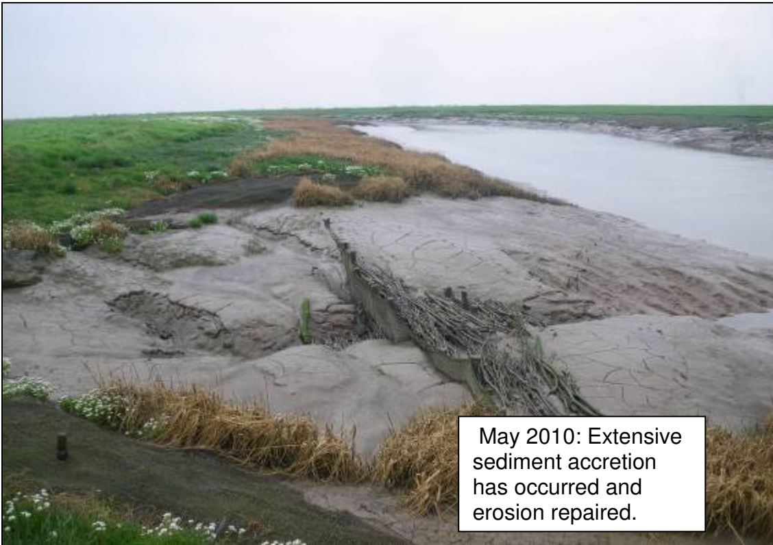
May 2010: The outfall is now completely protected from erosion
