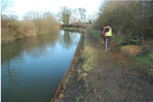
Early 2009 Structure completed
