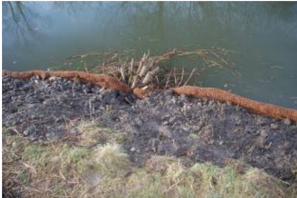
Early 2009 Small willow coppiced to allow access for works, New bank installed
