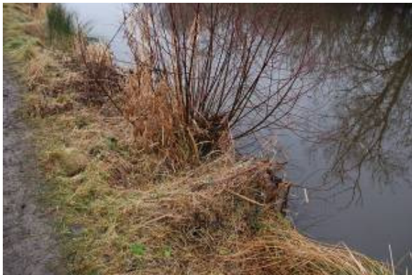
Early 2010 Willow re-growing and thick grasses and sedges covering structure
