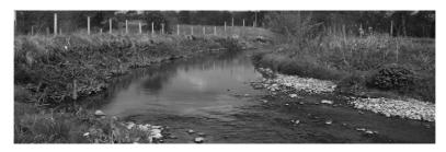
Plate 1 The test site (looking up stream) showing a bank side woody revetment in the River Manifold at Ludburn Farm in Staffordshire, UK
