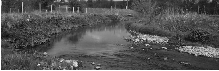
Plate 1 The test site (looking up stream) showing a bank side woody revetment in the River Manifold at Ludburn Farm in Staffordshire, UK
